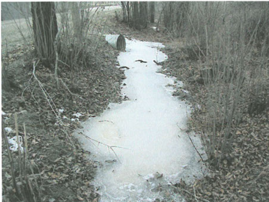
Photo: 8: Standing water at culvert inlet on centre slide, (Dec 05).
