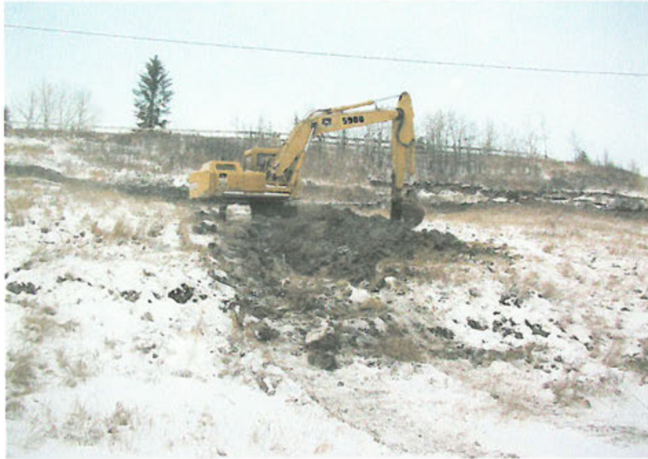
Photo 5: backfilling test pit on east slide, (Dec 05).
