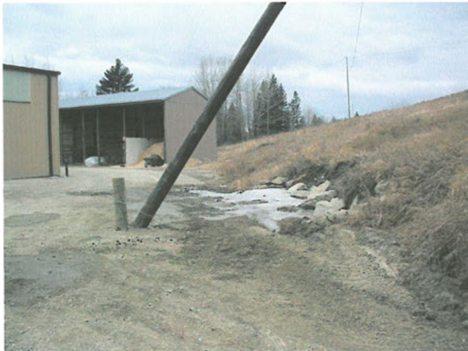
Photo 2: Ground water discharge forming ice sheet at base of east slide, (Nov 05).
