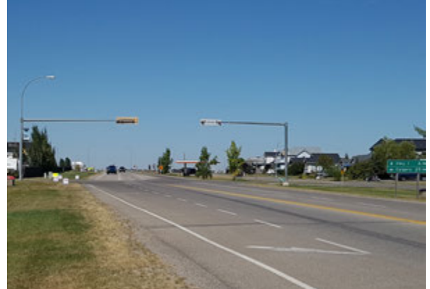
Crosswalks allow pedestrians to cross busy roadways such as this crossing of Centre Street in Langdon. Image: HDR
