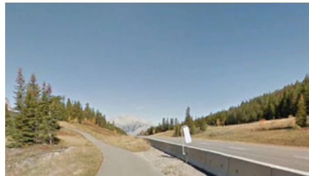
Example of a pathway that has a short section of steep grades because of a roadway cut (Legacy Trail, Banff National Park)
