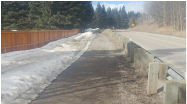
Some pathways are in their own right-of-way, while others are adjacent to roadways, like the West Bragg Creek Trail. Image: HDR
