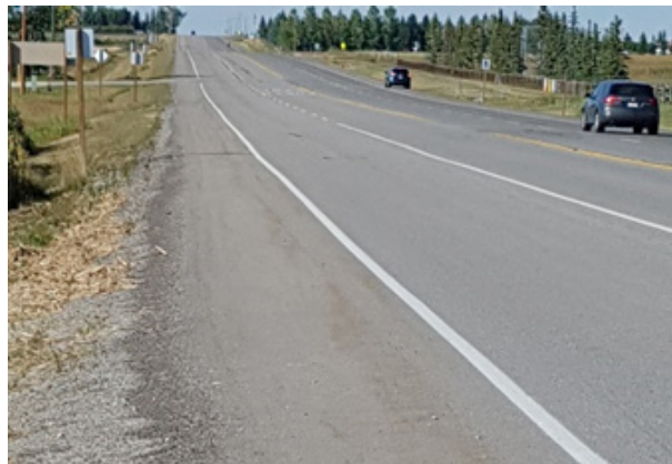
Paved shoulders are present on some roads in Rocky View County, like this example in Springbank. Image: HDR
