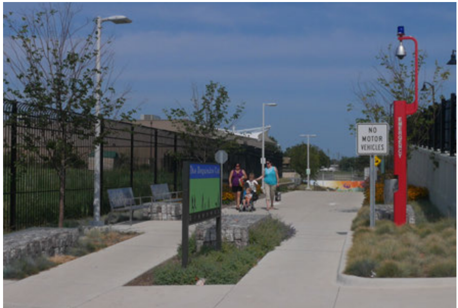
Figure 55: At path access points, the path can be configured as two 1.5 m (min) paths separated by a landscaped median. This example is in Detroit, MI, USA.
