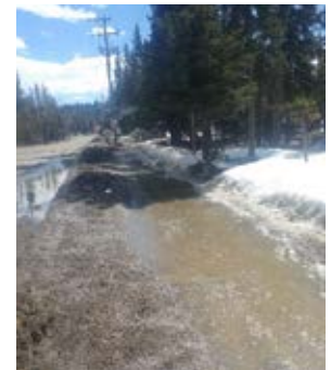
Existing pathway on Balsam Drive in Bragg Creek. Image: HDR
