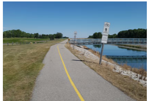
The WID Canal pathway is a shared-use pathway facility. Image: HDR
