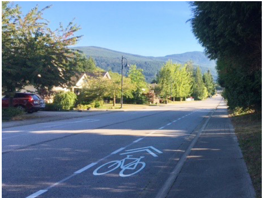
Figure 27: Advisory lane with shared lane markings in Gibsons, BC.
