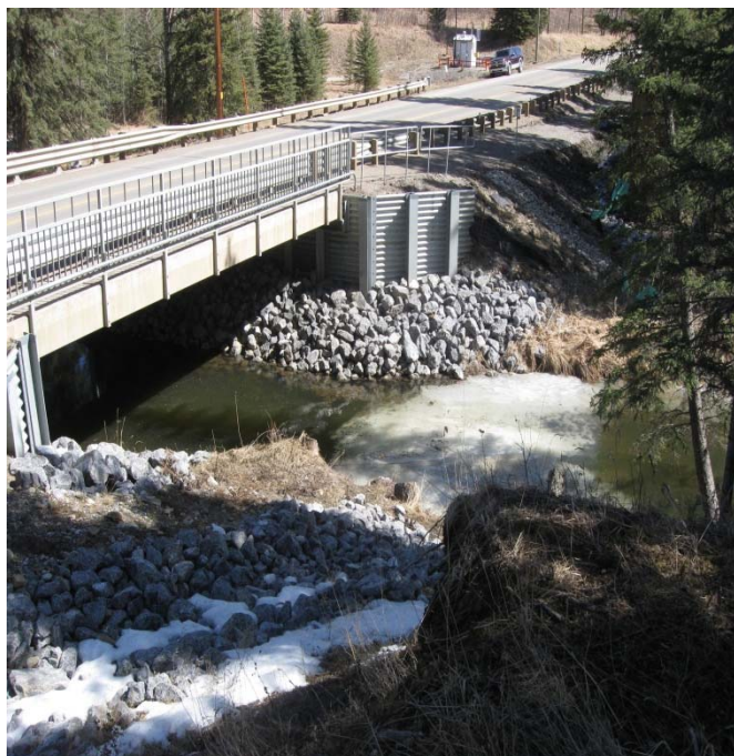
Bridge 1 across Bragg Creek
