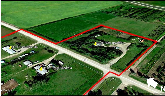
Figure 13: Development Cell A, Property Aerial
