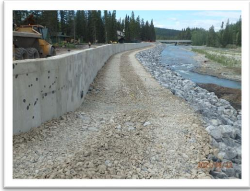
East Barrier: North of Balsam Bridge
