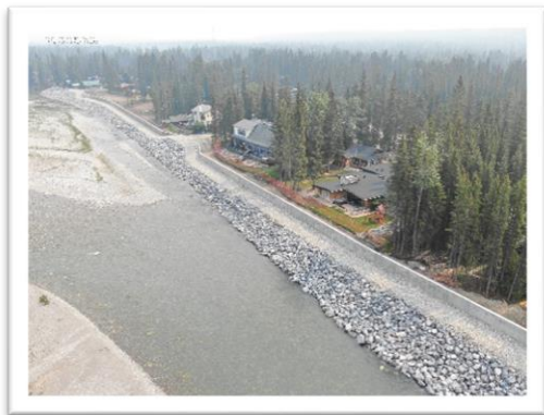
East Barrier: North of Balsam Bridge
