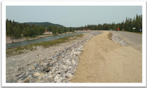
East Barrier – Hwy 22 Berm
