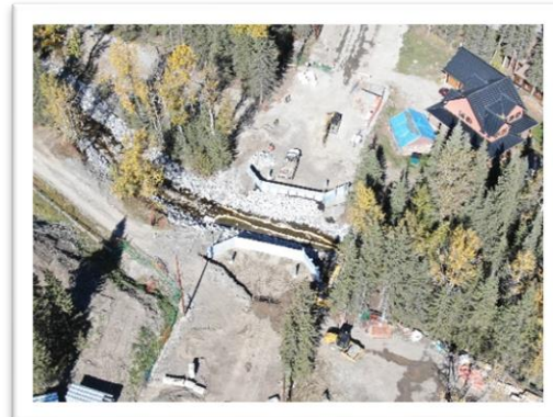
Bracken Bridge Replacement
