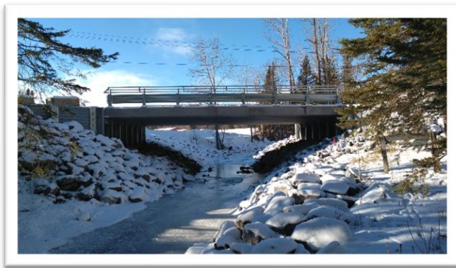
Bracken Bridge Constructed
