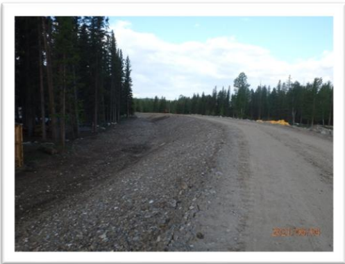
East Barrier - Berm
