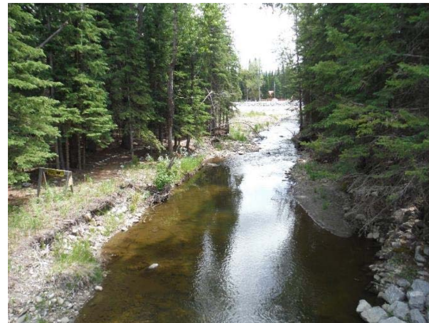
Photo 3 – Looking downstream from the Bracken Road Bridge. 22 June 2017
