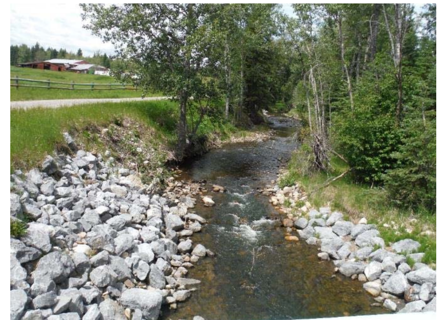
Photo 4 – Looking upstream from the Bracken Road Bridge. 22 June 2017
