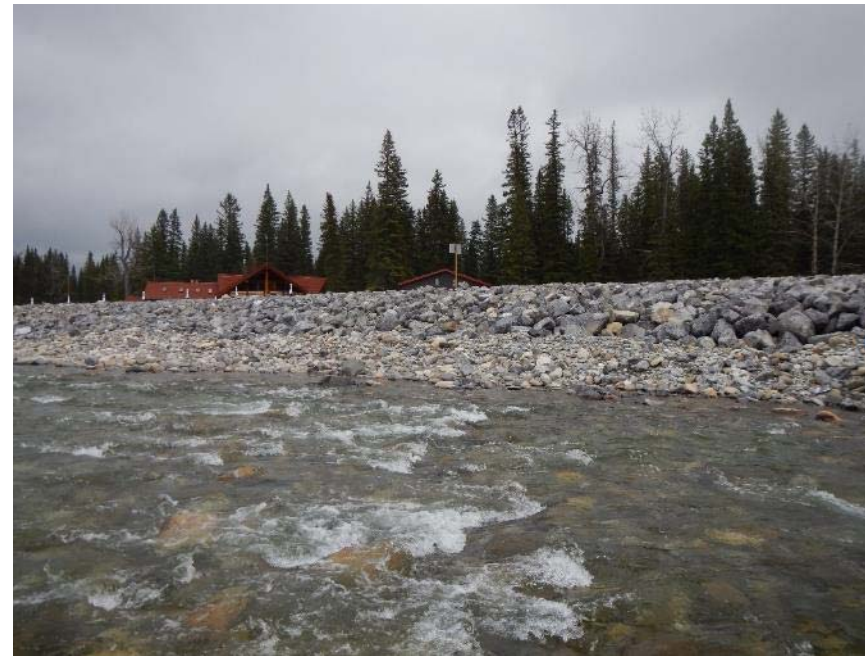
Photo 11: Existing riprap bank protection along the right bank extending past transects 11 and 12. 5 October 2016
