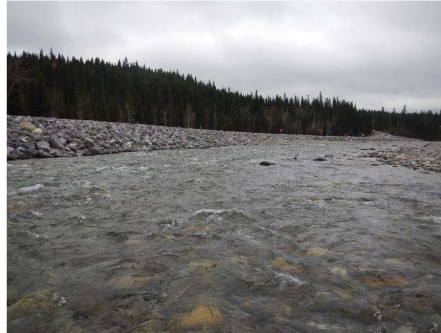
Photo 9: Looking upstream from transect 11 showing existing riprap bank protection 5 October 2016
