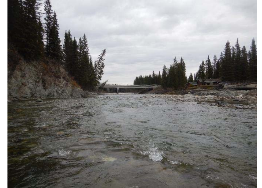
Photo 6: Looking downstream from transect 7 showing large bedrock outcrop along the right bank and the Balsam Ave Bridge in the distance. 5 October 2016
