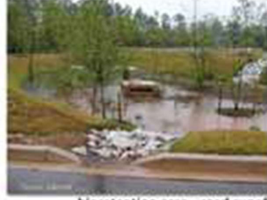
bioretention area - road runoff
