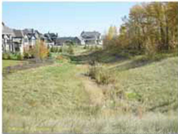
bioswale - lot runoff post establishment
