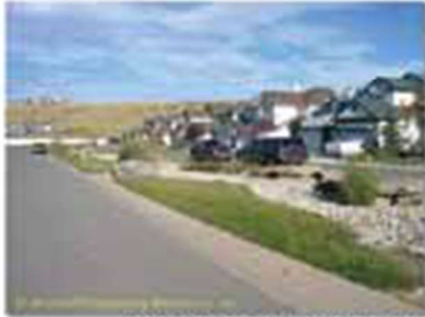
bioretention area - road runoff
