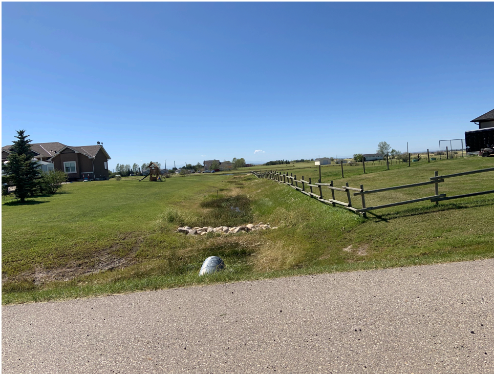
Drainage swales in the existing country residential community to the south
