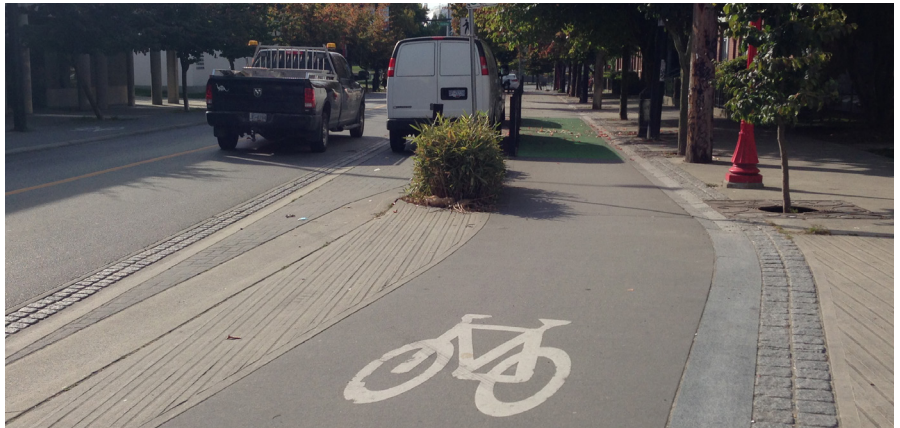
Figure 23: Bicycle pavement marking, textured delineation, tree buffer space, and varying materials distinguish the protected bicycle lane from the sidewalk in Vancouver, BC.
