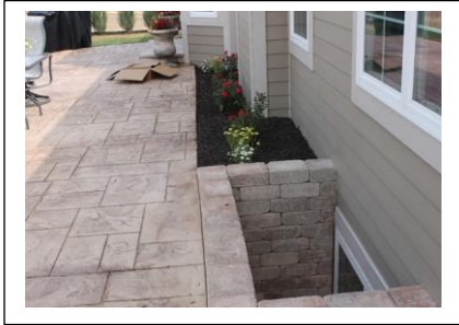
Guard NOT Required Window well adjacent to landscaping
