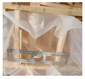
Example of a mounting plate for a Can-less style recessed light installed in a ceiling with a polyethylene sheet cover, which will be sealed to the polyethylene at the ceiling
