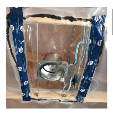
Example of a Can style IC rated recessed light housing installed in a ceiling with a poly hat, and sealed to the adjacent polyethylene.
