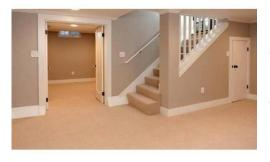
Handrail required on one side throughout flight of stair. Where the bottom open side is less than 600 mm to floor level, no guardrail is required.
