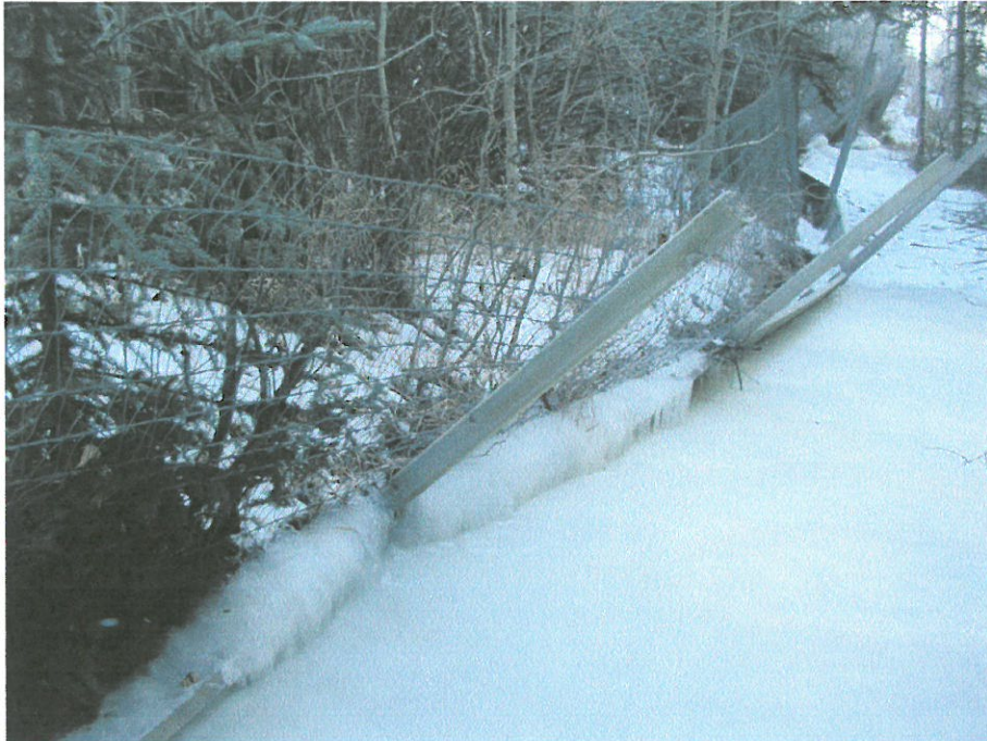
Photo 9: View of ice formed by heavy ground water discharge along toe of centre slide. Note tilted fence posts from slide movement, (Dec 05).
