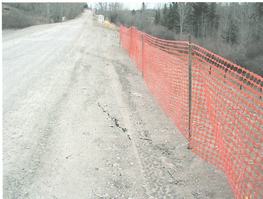
Photo 10: Looking east along top of west slide. Open tension crack visible along edge of roadway, (Nov 05).
