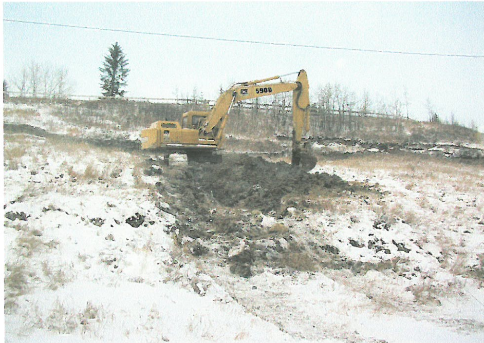
Photo 5: backfilling test pit on east slide, (Dec 05).
