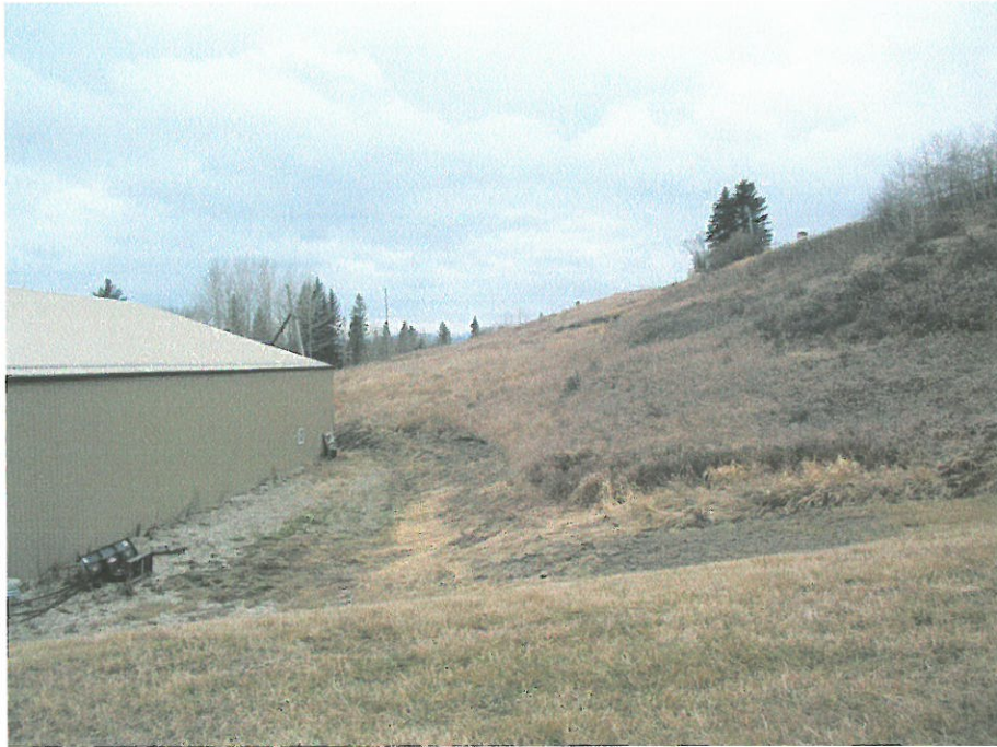
Photo 1: View looking west over east slide, showing narrow gap between base of slope and barn and slide scarp on below bushes on upper slope, (Nov 05).
