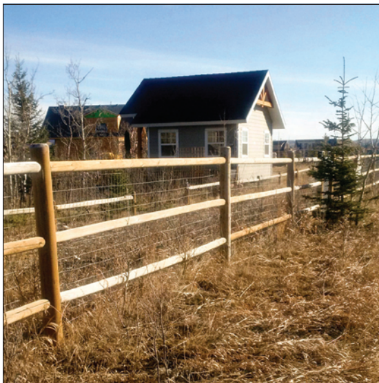
Adding wire mesh to a decorative fence will provide a barrier for pets and livestock.
