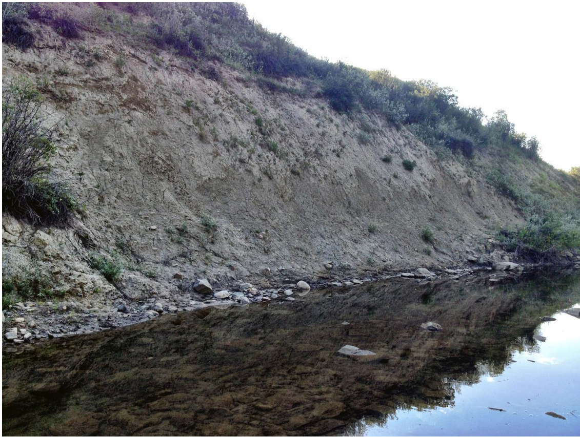
Photo 16. Riparian area with potential for erosion
