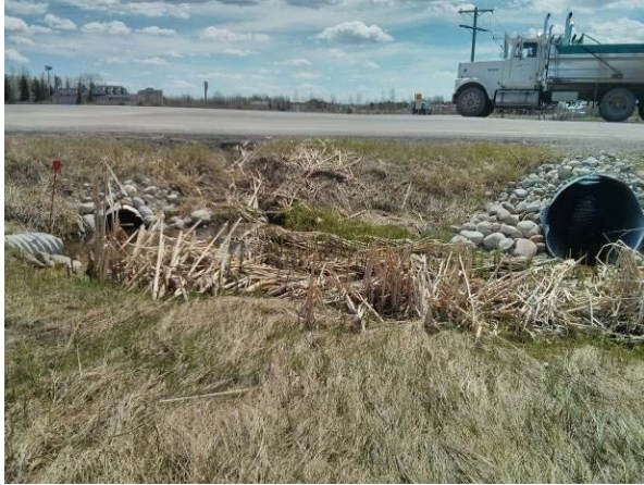
SC-28-4 Upstream Facing South
