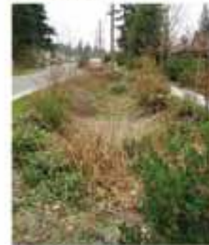
bioswale - road runoff
