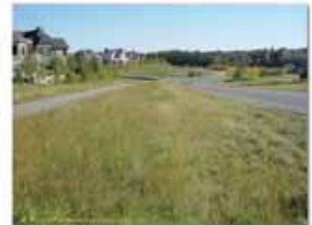
bioswale - road runoff
