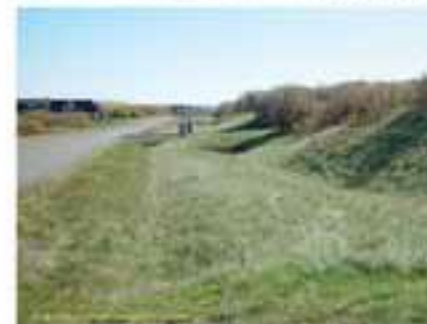
bioswale - road runoff
